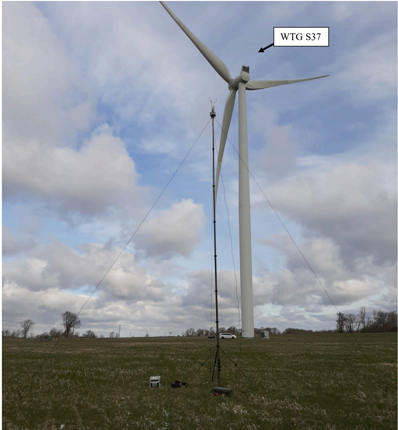
Meteorological Tower Location – April 22, 2021
