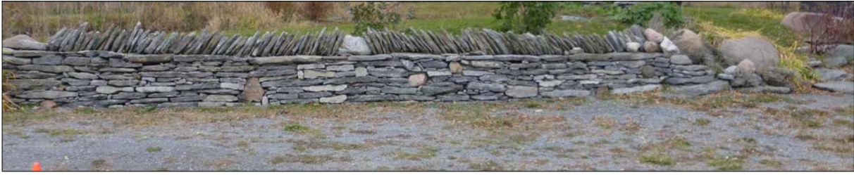
Dry Stone Fence Photo - Section 4 - 0m to 5m
