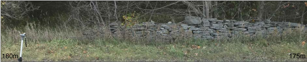
Dry Stone Fence Photo - 175m to 180m
