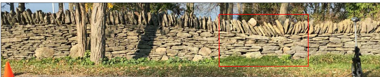
Dry Stone Fence Photo - 25m to 30m
