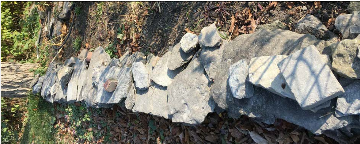
Dry Stone Fence Photo - 10m to 15m
