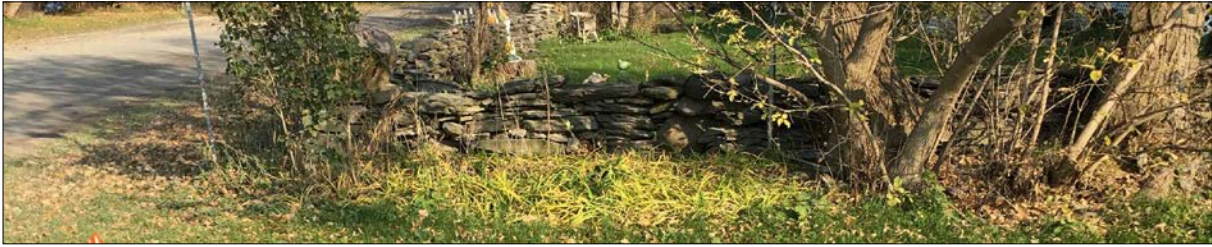
Dry Stone Fence Photo - Section 2 - 0m to 5m
