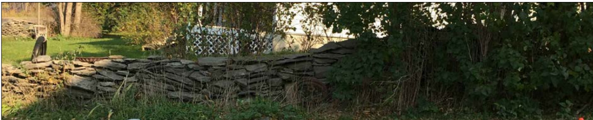
Dry Stone Fence Photo - Section 2 - 10m to 15m
