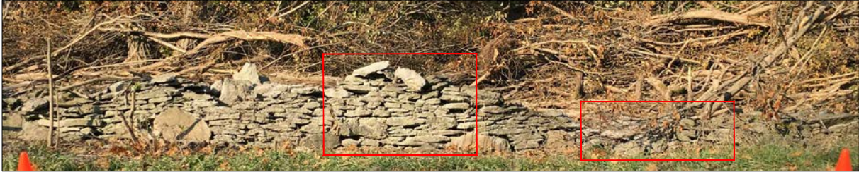
Dry Stone Fence Photo - 135m to 140m
