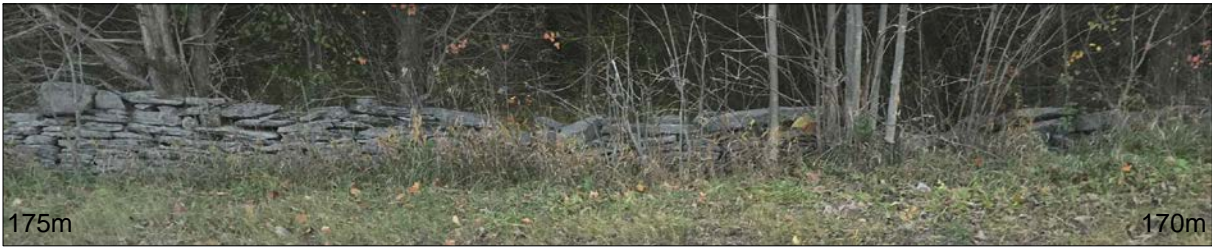
Dry Stone Fence Photo - 170m to 175m
