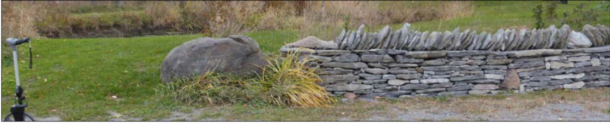
Dry Stone Fence Photo - Section 4 - 5m to 8.5m
