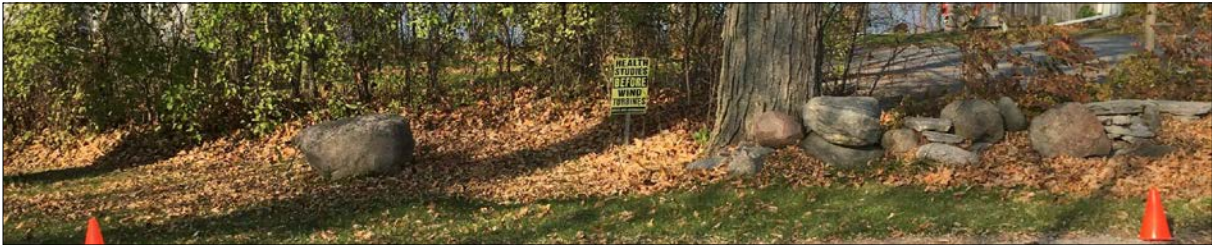
Dry Stone Fence Photo - 0m to 5m
