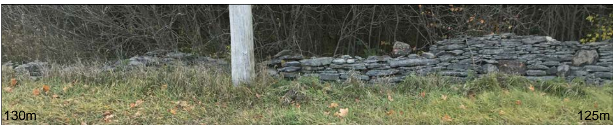
Dry Stone Fence Photo - 125m to 130m
