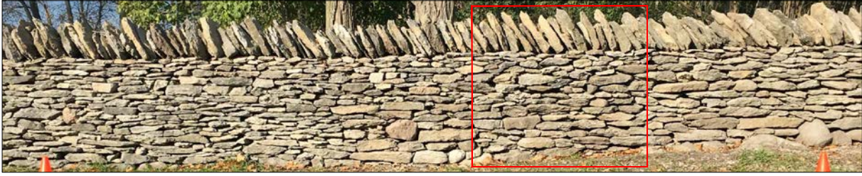
Dry Stone Fence Photo - 95m to 100m
