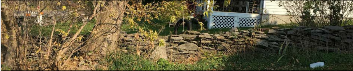
Dry Stone Fence Photo - Section 2 - 5m to 10m
