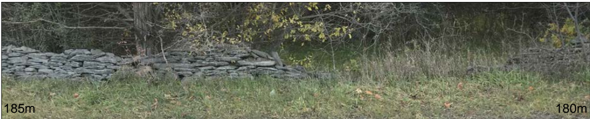
Dry Stone Fence Photo - 180m to 185m
