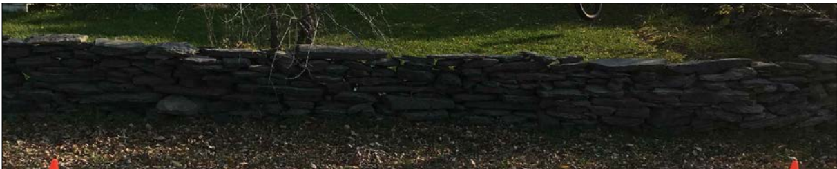
Dry Stone Fence Photo - Section 1 - 20m to 25m
