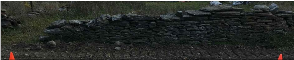
Dry Stone Fence Photo - 0m to 5m
