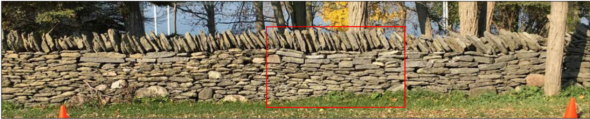
Dry Stone Fence Photo - 15m to 20m
