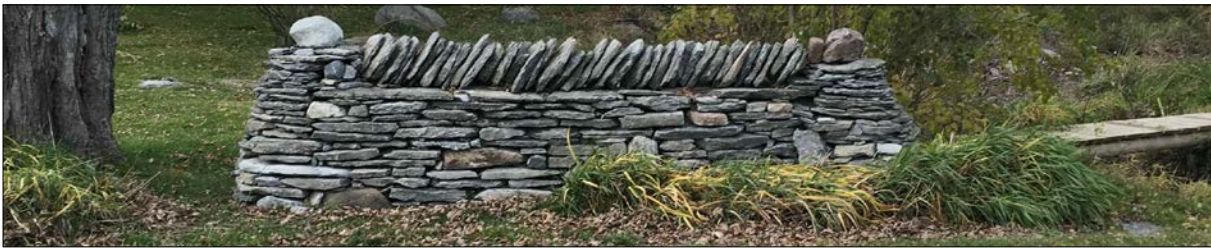
Dry Stone Fence Photo - Section 1 - 0m to 4.75m
