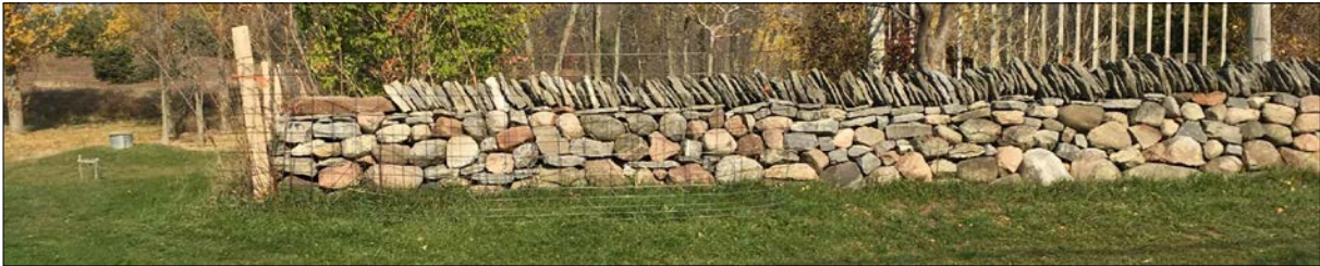
Dry Stone Fence Photo - 0m to 5m
