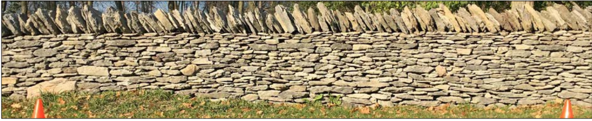
Dry Stone Fence Photo - 90m to 95m
