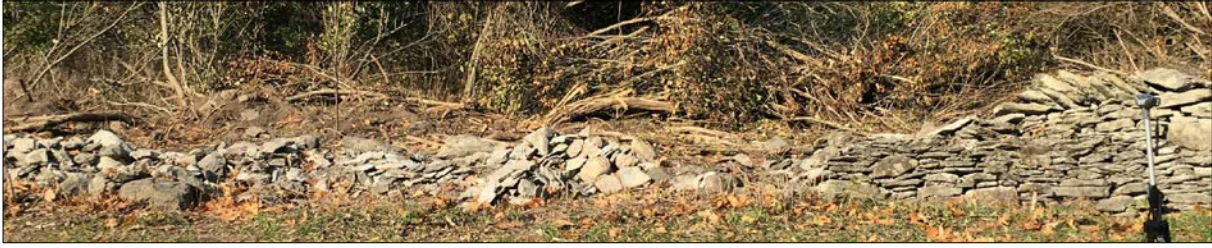
Dry Stone Fence Photo - 115m to 120m
