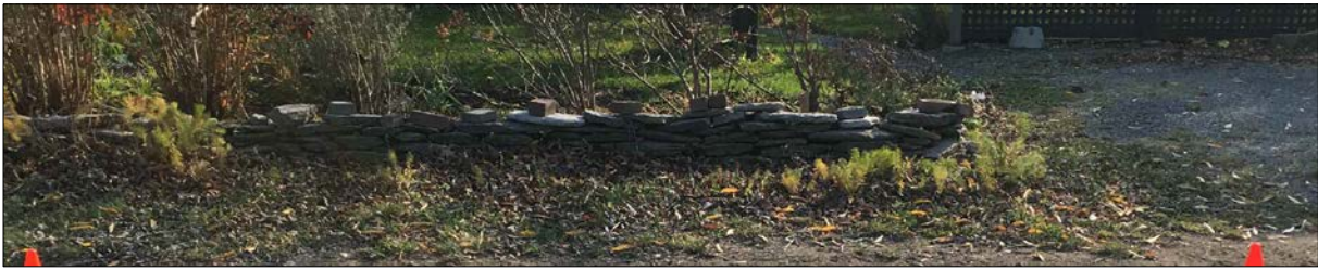
Dry Stone Fence Photo - 10m to 15m
