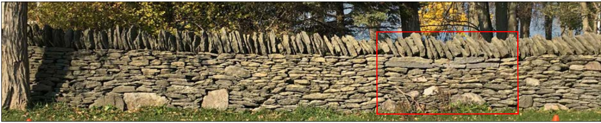
Dry Stone Fence Photo - 10m to 15m
