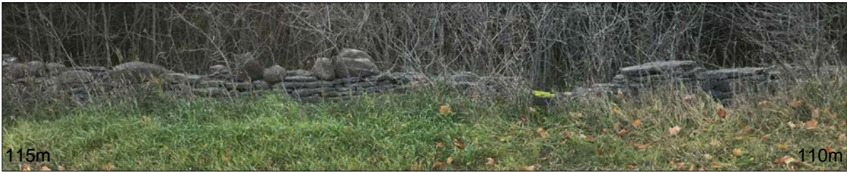
Dry Stone Fence Photo - 110m to 115m
