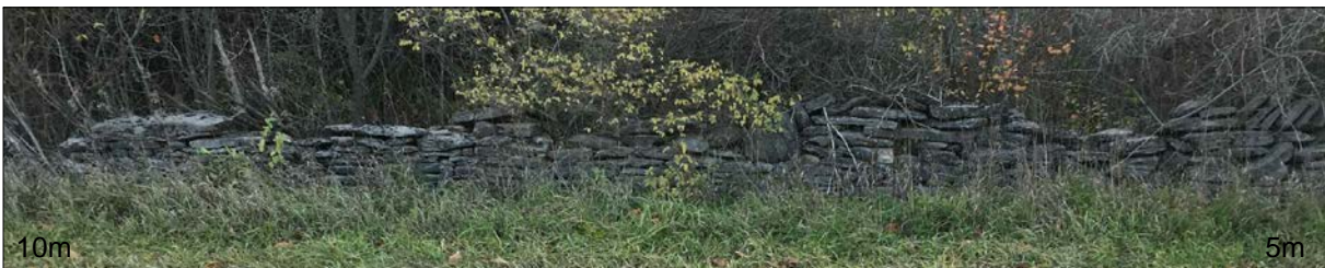
Dry Stone Fence Photo - 5m to 10m
