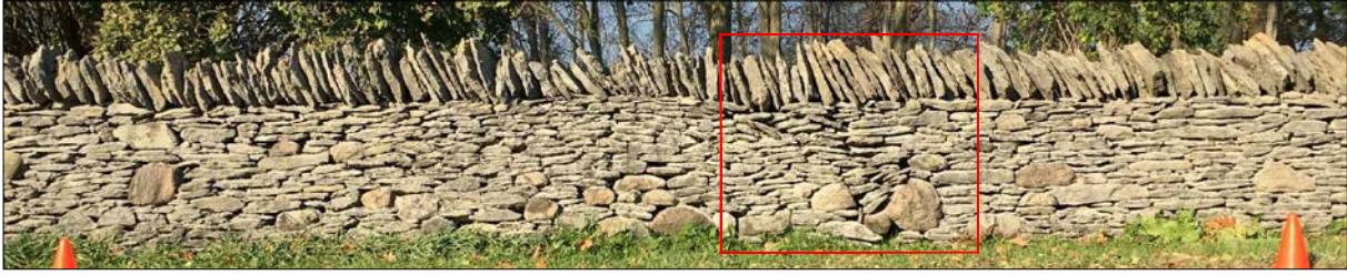
Dry Stone Fence Photo - 75m to 80m
