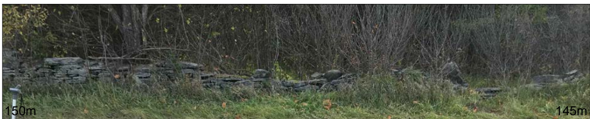
Dry Stone Fence Photo - 145m to 150m
