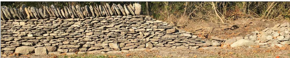
Dry Stone Fence Photo - 105m to 110m
