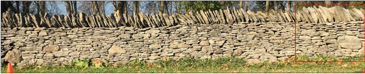
Dry Stone Fence Photo - 80m to 85m
