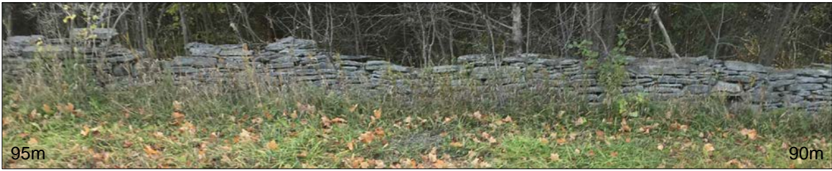
Dry Stone Fence Photo - 90m to 95m
