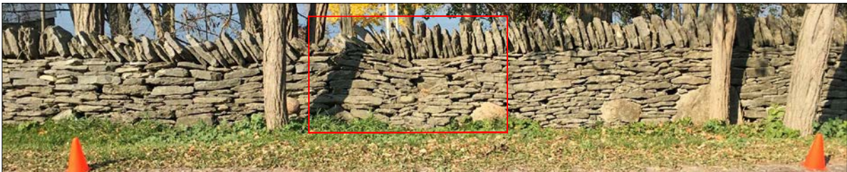
Dry Stone Fence Photo - 20m to 25m
