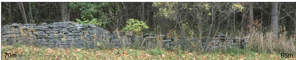
Dry Stone Fence Photo - 65m to 70m
