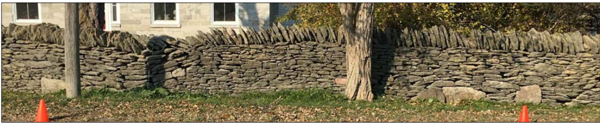
Dry Stone Fence Photo - 5m to 10m
