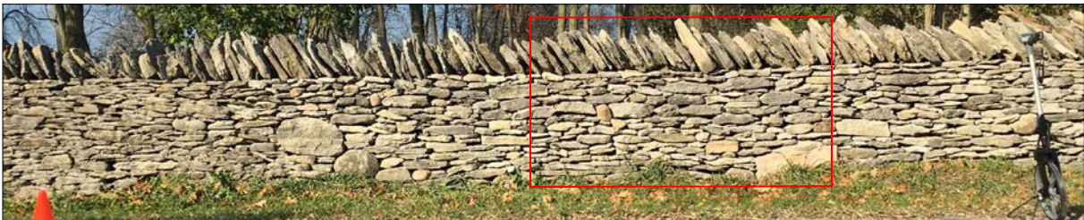
Dry Stone Fence Photo - 85m to 90m
