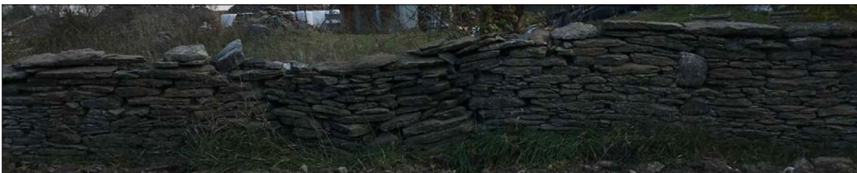
Dry Stone Fence Photo - 5m to 10m
