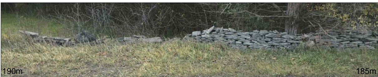
Dry Stone Fence Photo - 185m to 190m
