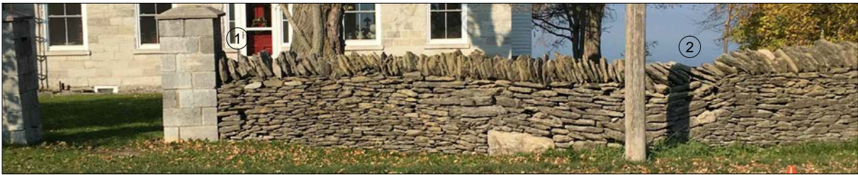
Dry Stone Fence Photo - 0m to 5m
