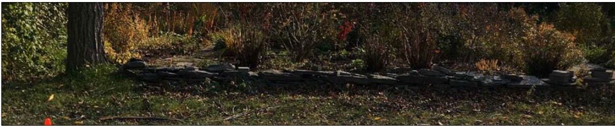
Dry Stone Fence Photo - 0m to 5m
