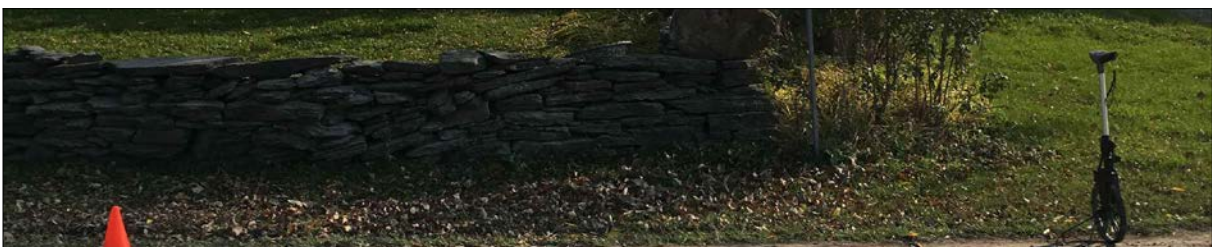
Dry Stone Fence Photo - Section 1 - 25m to 30m
