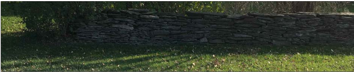
Dry Stone Fence Photo - Section 1 - 0m to 5m
