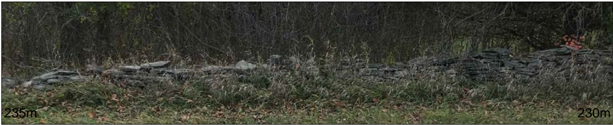
Dry Stone Fence Photo - 230m to 235m
