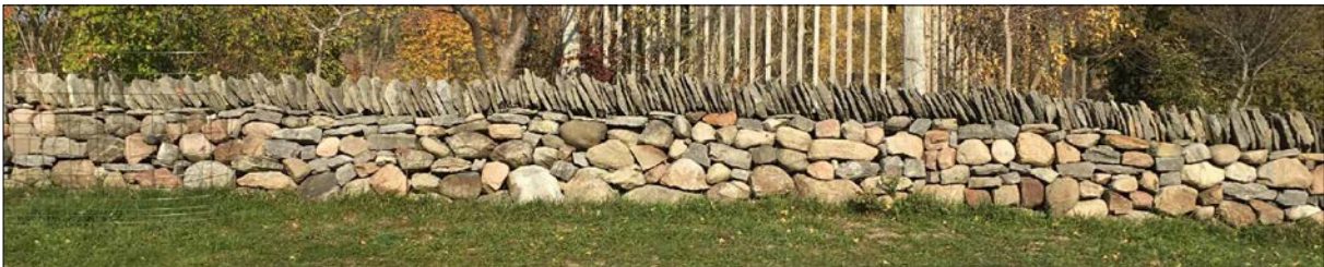
Dry Stone Fence Photo - 5m to 10m
