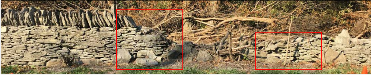
Dry Stone Fence Photo - 130m to 135m
