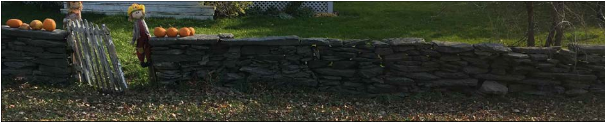
Dry Stone Fence Photo - Section 1 - 15m to 20m
