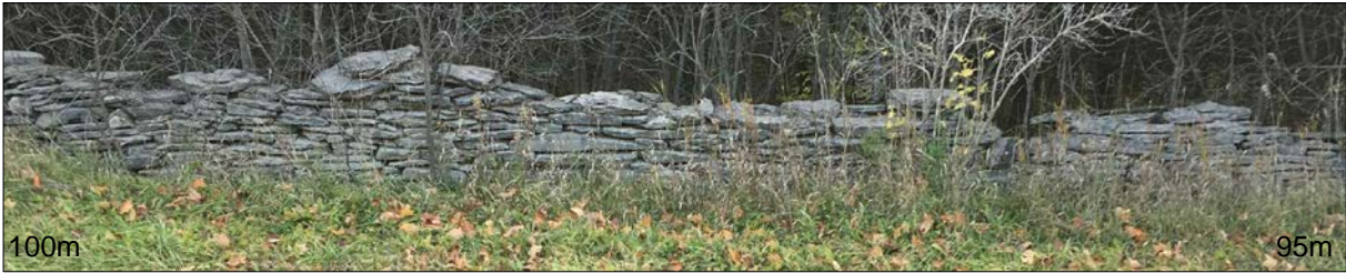
Dry Stone Fence Photo - 95m to 100m
