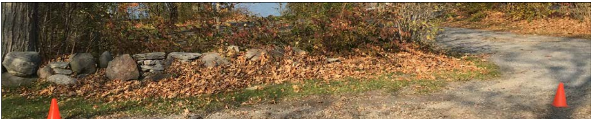
Dry Stone Fence Photo - 3m to 8m
