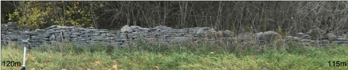
Dry Stone Fence Photo - 115m to 120m
