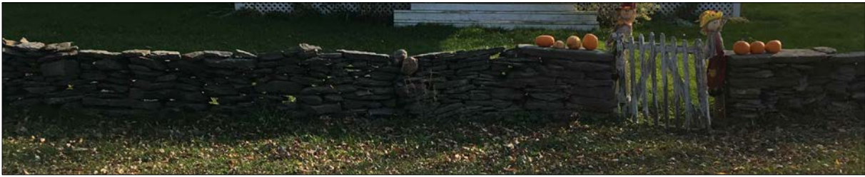
Dry Stone Fence Photo - Section 1 - 10m to 15m
