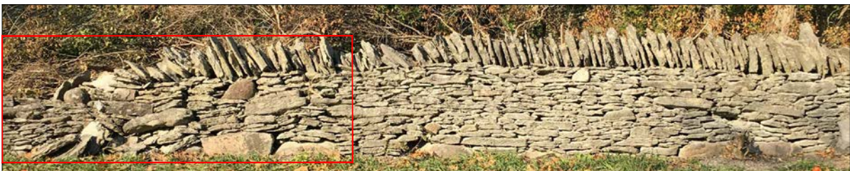
Dry Stone Fence Photo - 125m to 130m
