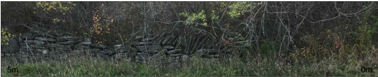
Dry Stone Fence Photo - 0m to 5m
