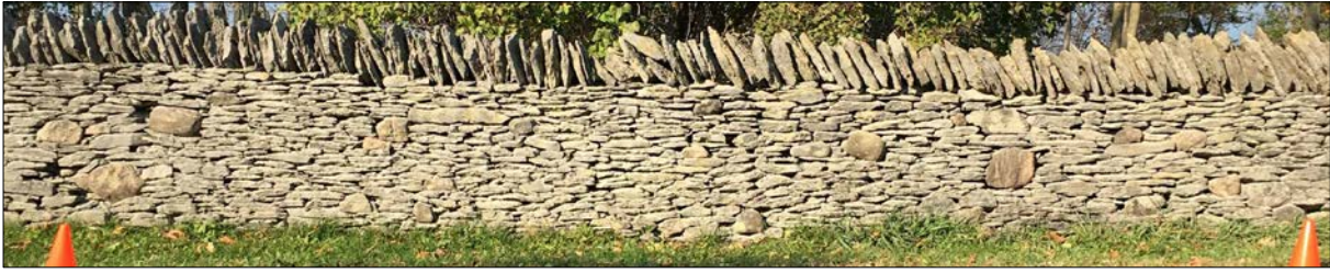
Dry Stone Fence Photo - 70m to 75m
