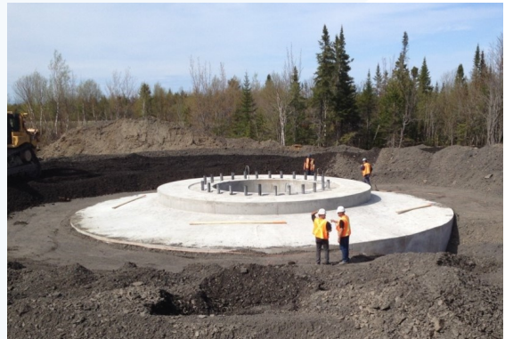
Concrete Placement/Curing
