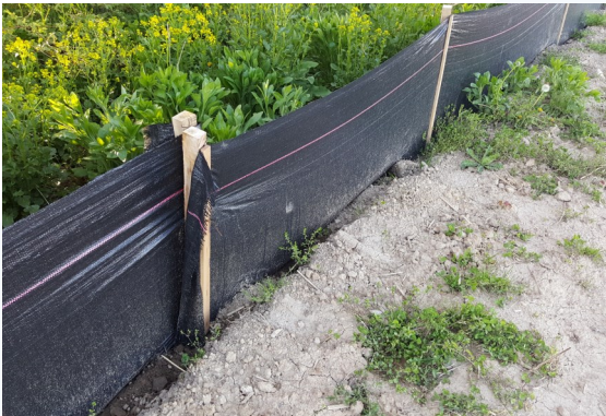
Sediment Erosion Control: Silt Fence
