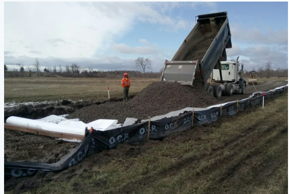
Road Construction (Strip, Geotextile, Material Placement)
