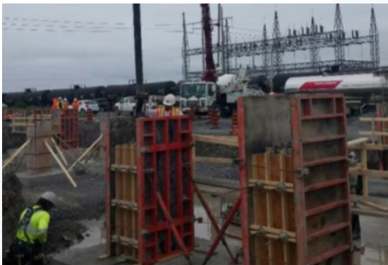
Concrete Placement (For Structures)
