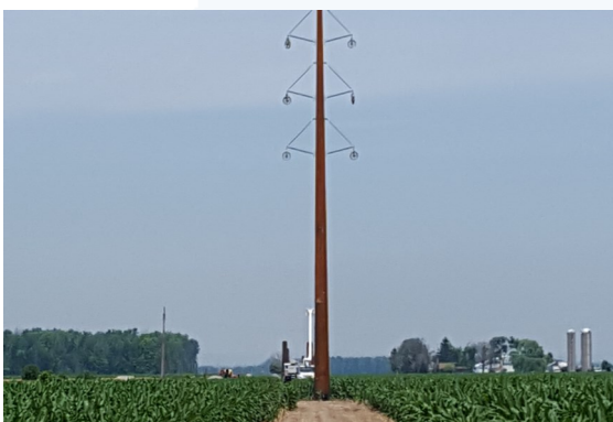
Transmission Pole Erection
