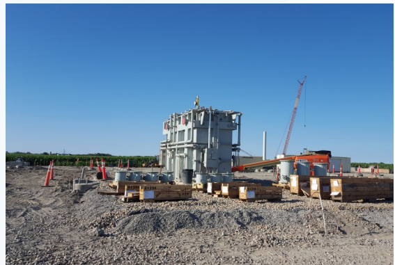
Equipment Delivery & Installation
