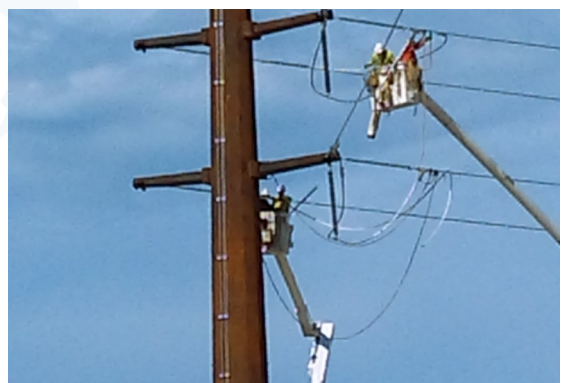
Wiring (Substation & Transmission Line Stringing)
