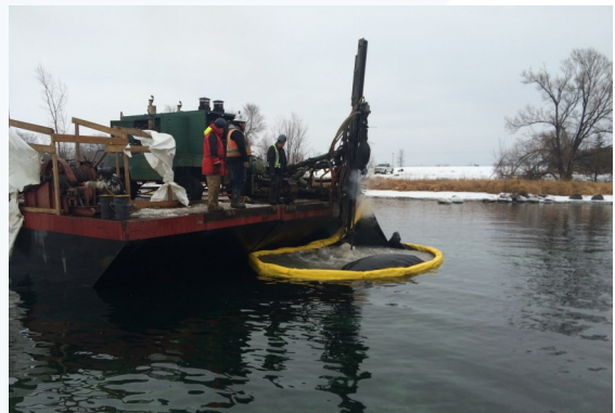
Pile Drilling
