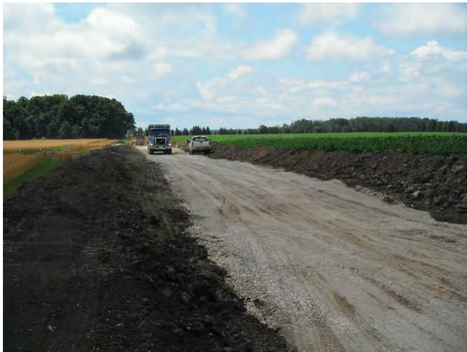
Figure 10 Typical access road construction at a wind project
