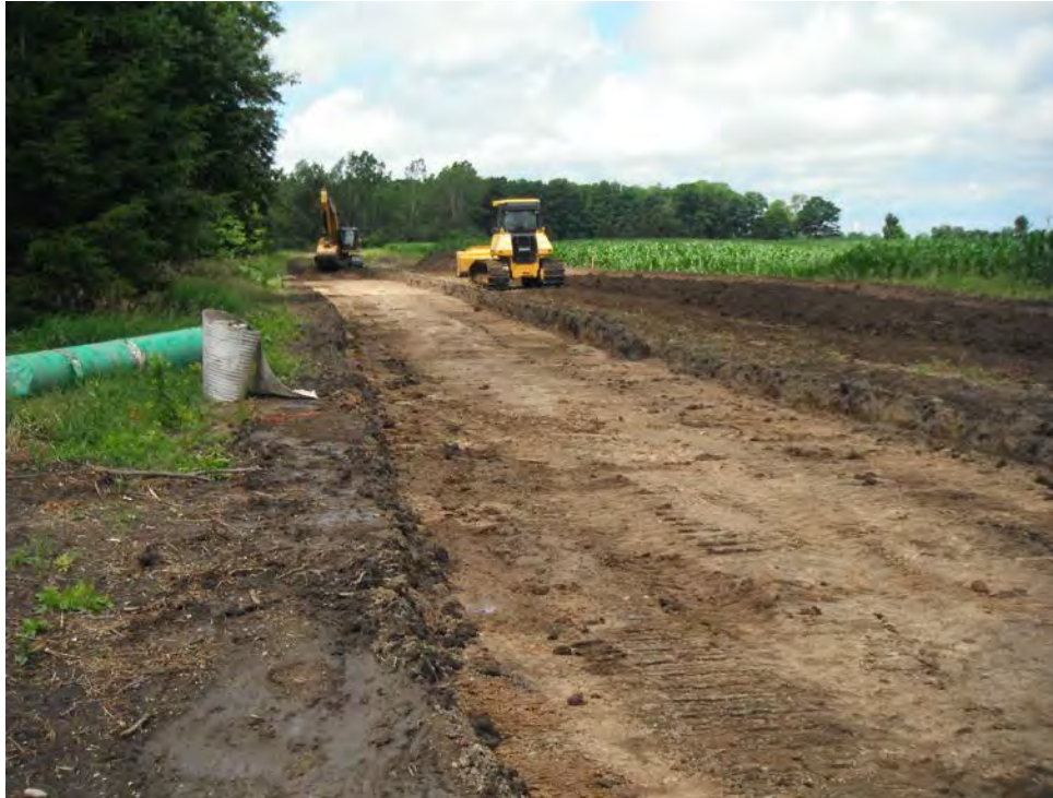
Figure 9 Typical access road construction at a wind project
