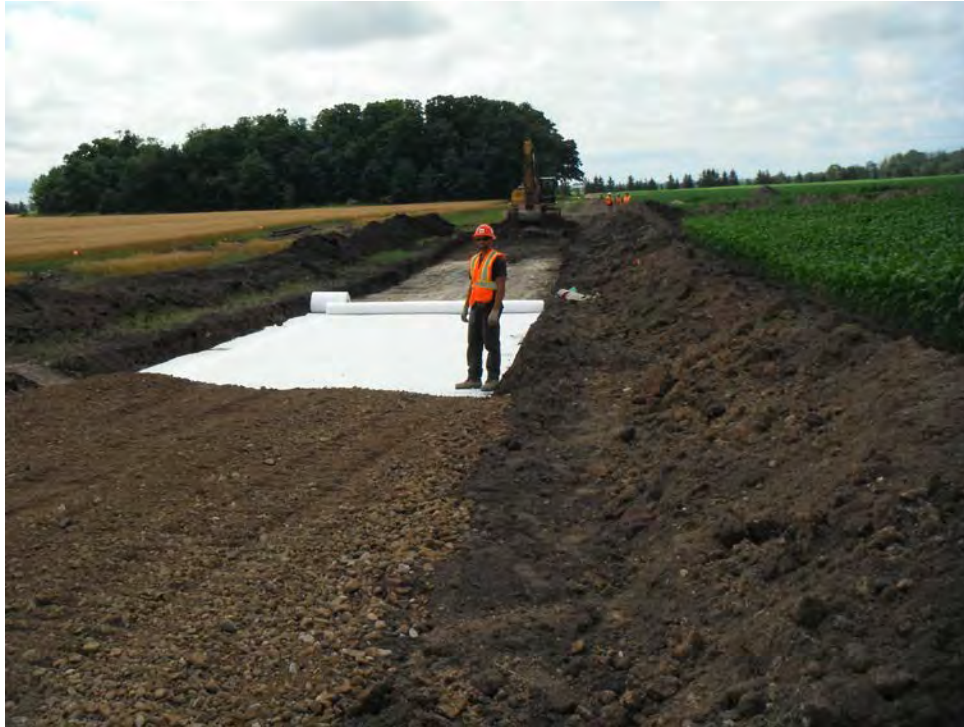
Figure 11 Typical access road construction at a wind project
