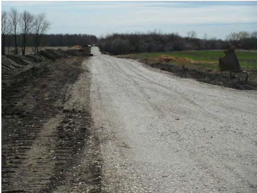
Figure 7 Typical access road construction at a wind project
