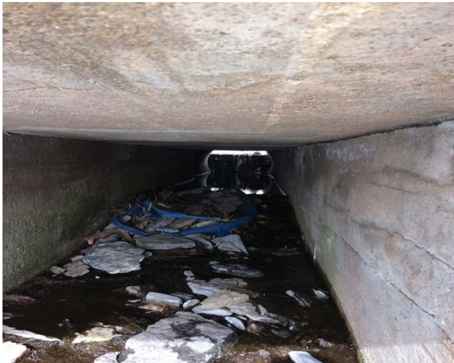
NORTH WALL BASE, WEST ELEVATION EROSION AND LACK OF FOUNDATION BOND
