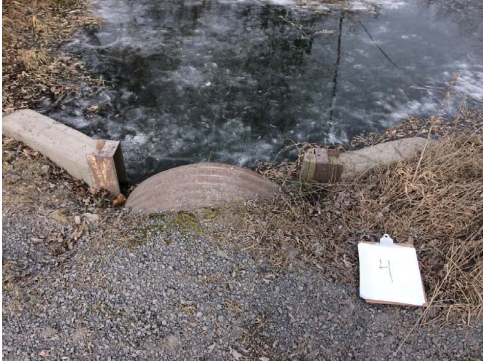
INLET LOOKING WEST
