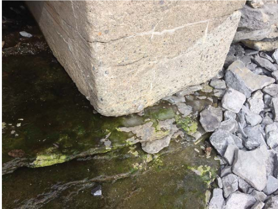
NORTH WALL BASE, WEST ELEVATION EROSION AND LACK OF FOUNDATION BOND
