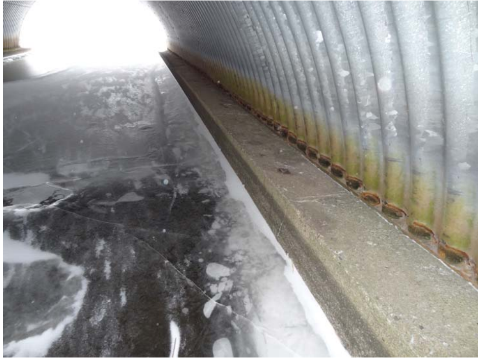
CONCRETE FOOTING AND CONNECTION POINTS
