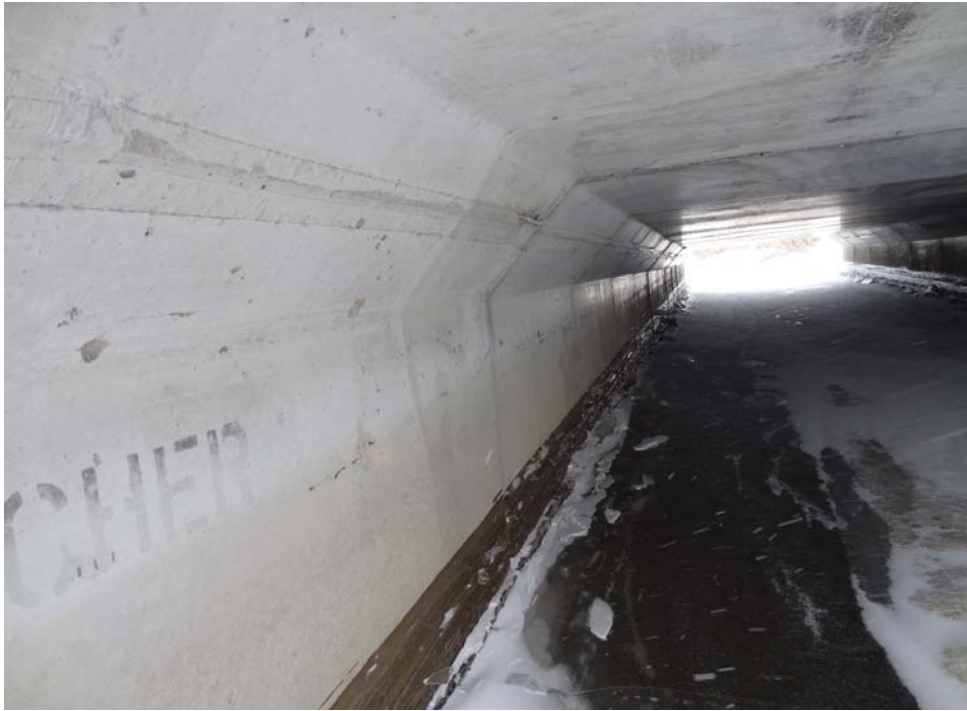
SOUTHEAST END SECTION OF PRE-CAST CULVERT BARREL
