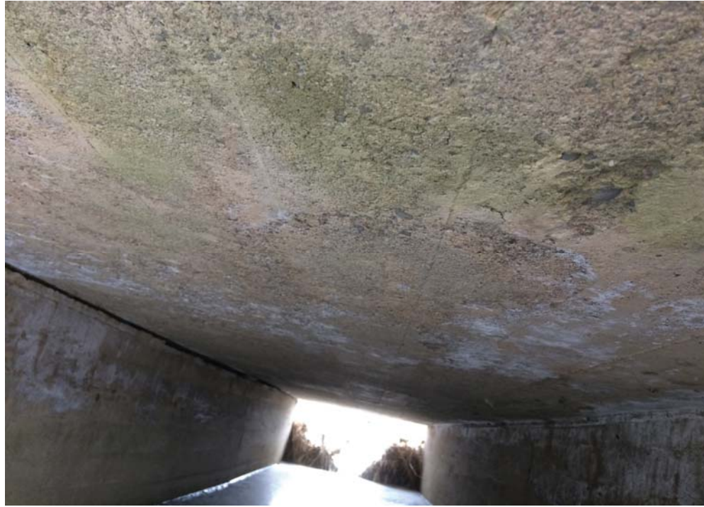
EAST ELEVATION, CULVERT BARREL
