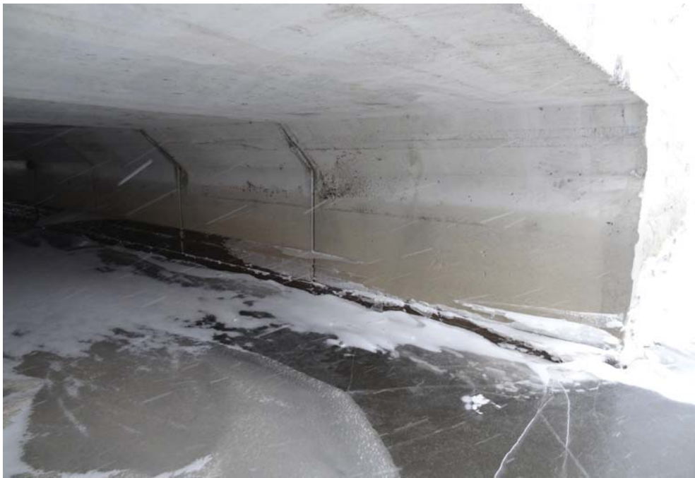
SOUTH WEST END SECTION OF PRE-CAST CULVERT BARREL
