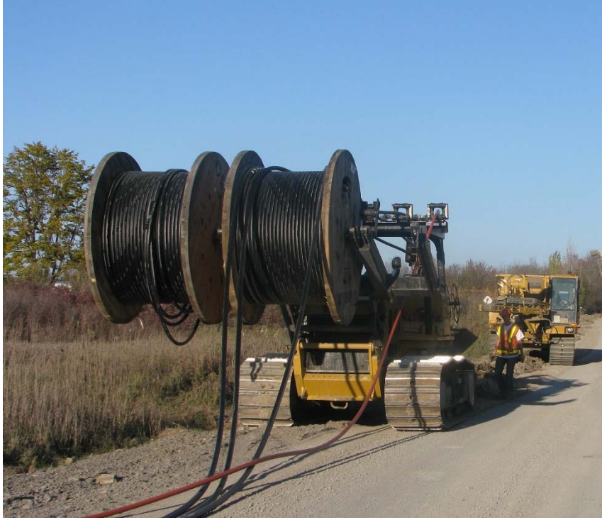
Figure 7 - Trenching and Cable Placement
