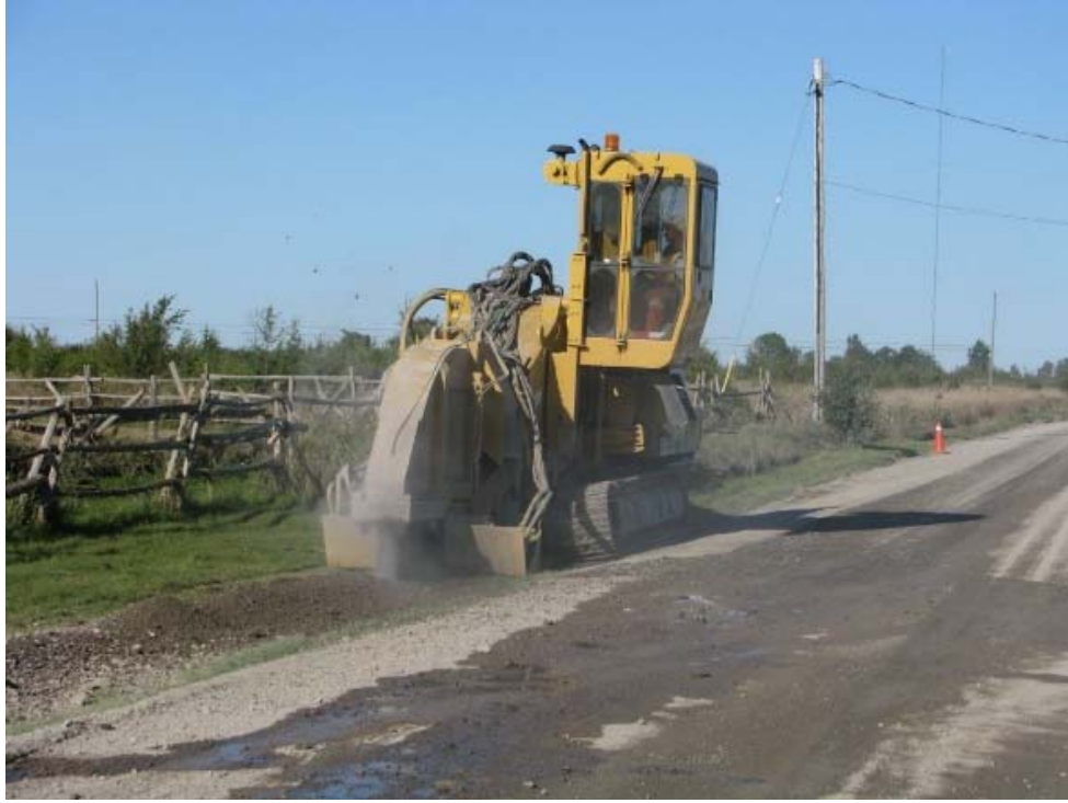
Figure 5 – Trenching Operations
