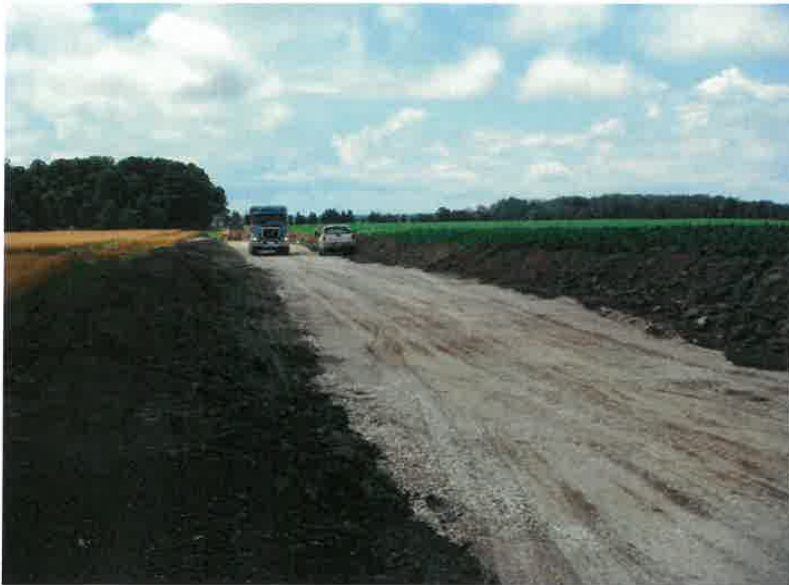
Photo 4 Typical access road construction at a wind project
