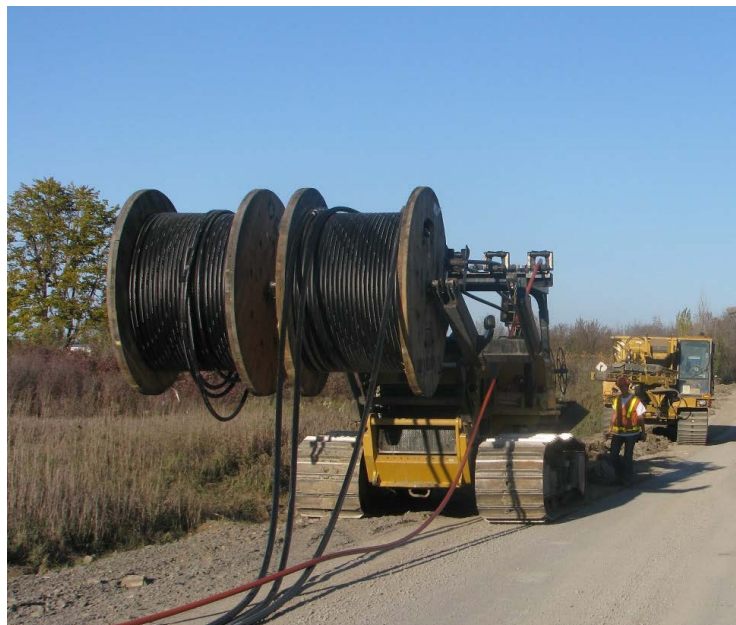
Figure 6 - Trenching and Cable Placement
