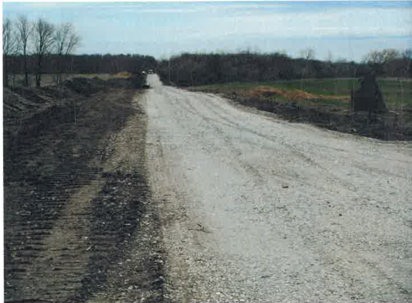
Photo 1 Typical access road construction at a wind project
