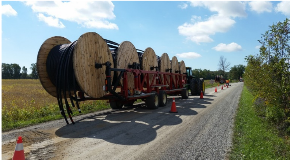
Figure 5 - Cable Spool Trailer
