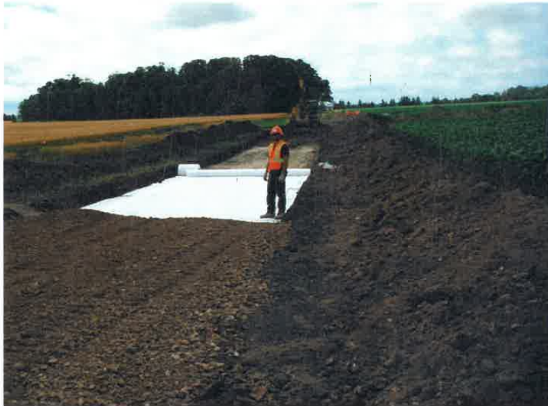
Photo 5 Typical access road construction at a wind project
