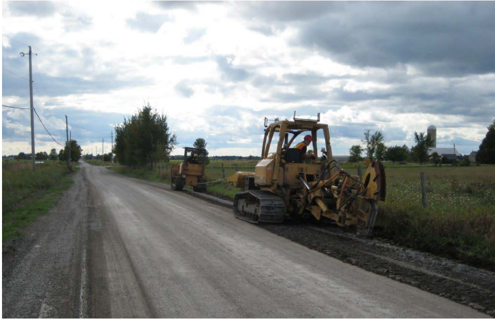
Figure 7 - Roadside Plowing
