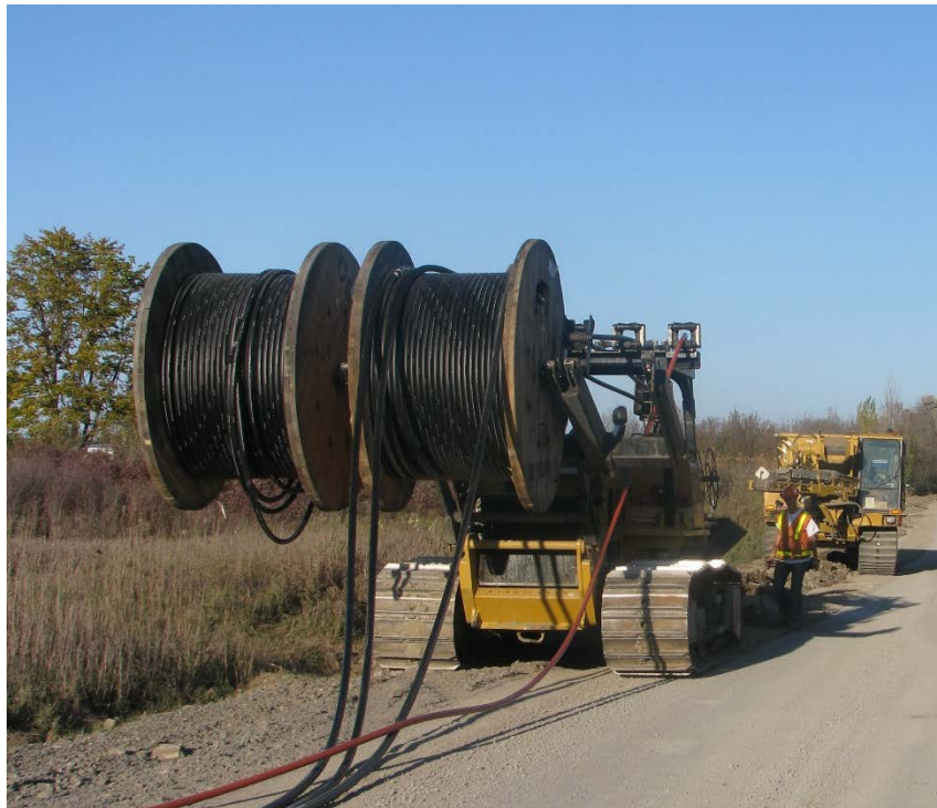
Figure 6 - Trenching and Cable Placement
