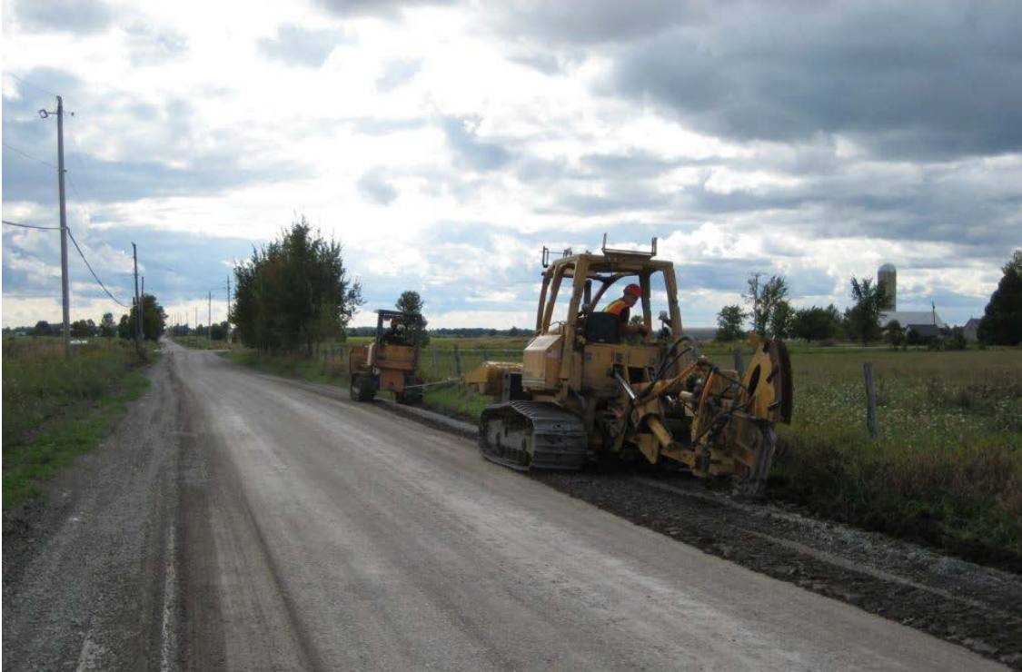
Figure 7 - Roadside Plowing
