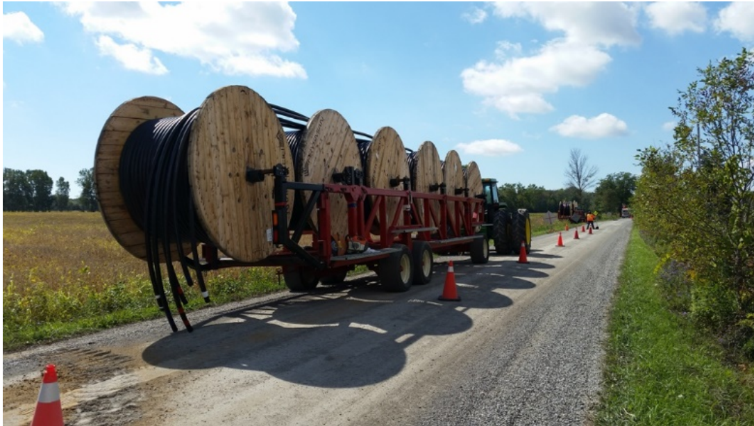
Figure 5 - Cable Spool Trailer
