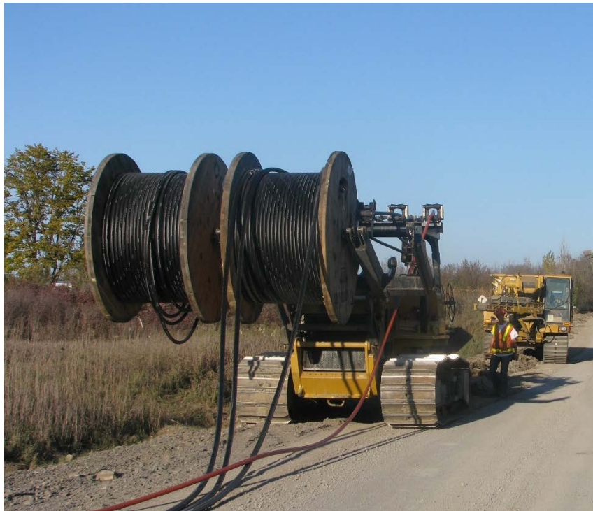
Figure 6 - Trenching and Cable Placement
