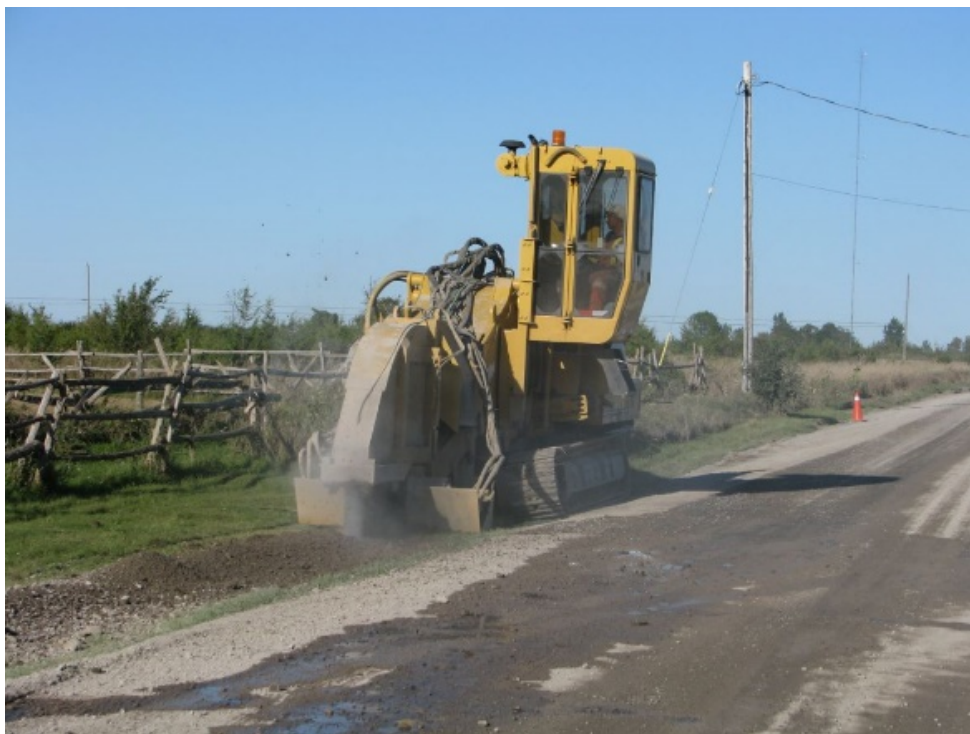
Figure 4 – Trenching Operations
