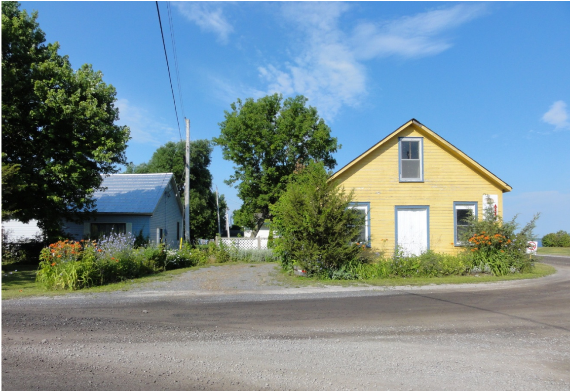
Plate 23: Front elevation of 20 Emerald 40 Foot Road, BHR 17
