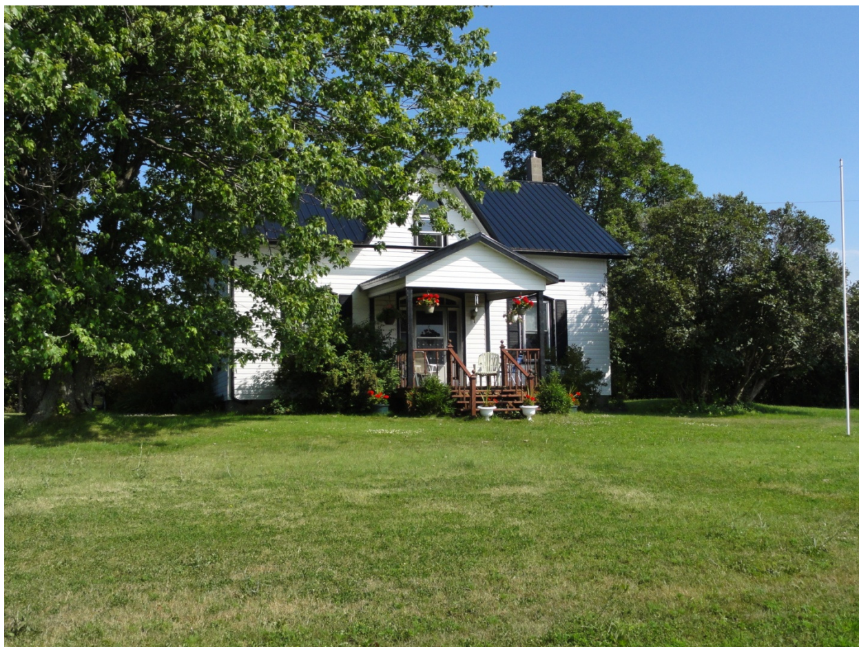
Plate 32: 5950 Second Concession Road, BHR 21
