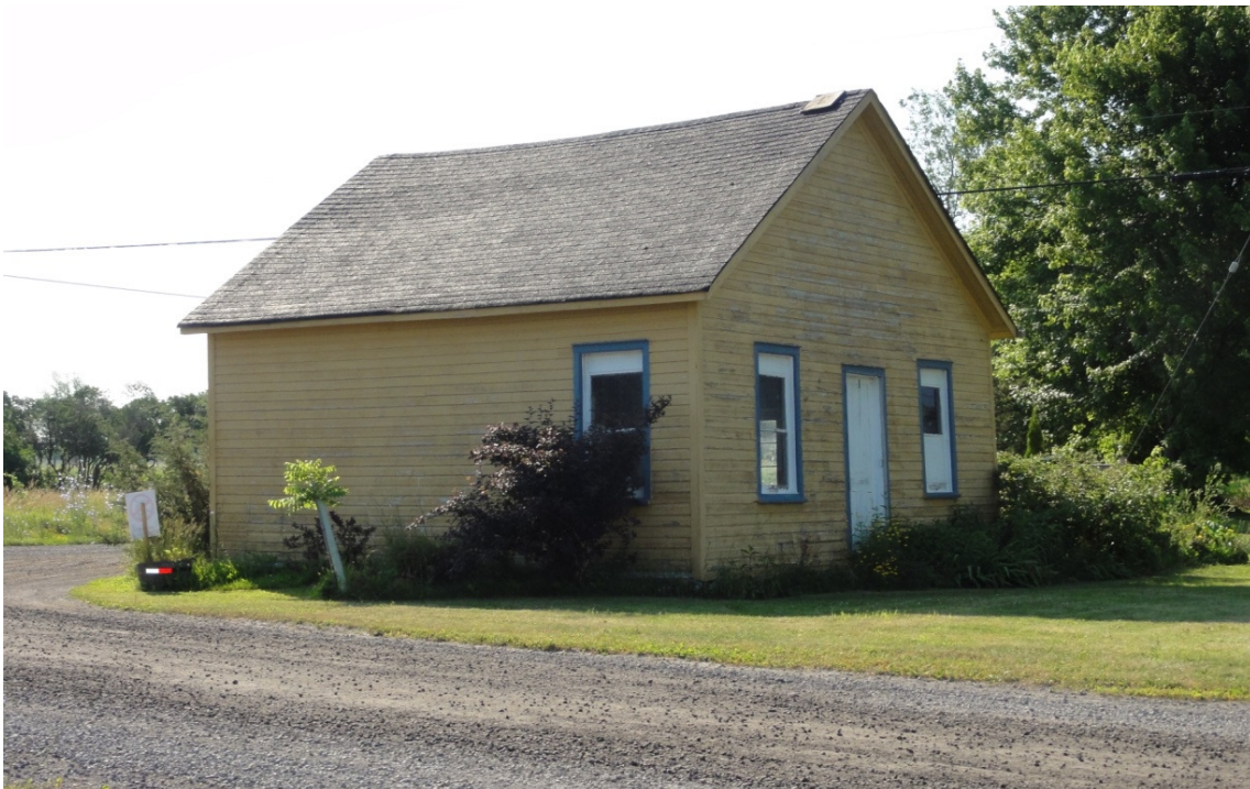
Plate 24: Rear Elevation of 20 Emerald 40 Foot Road, BHR 17
