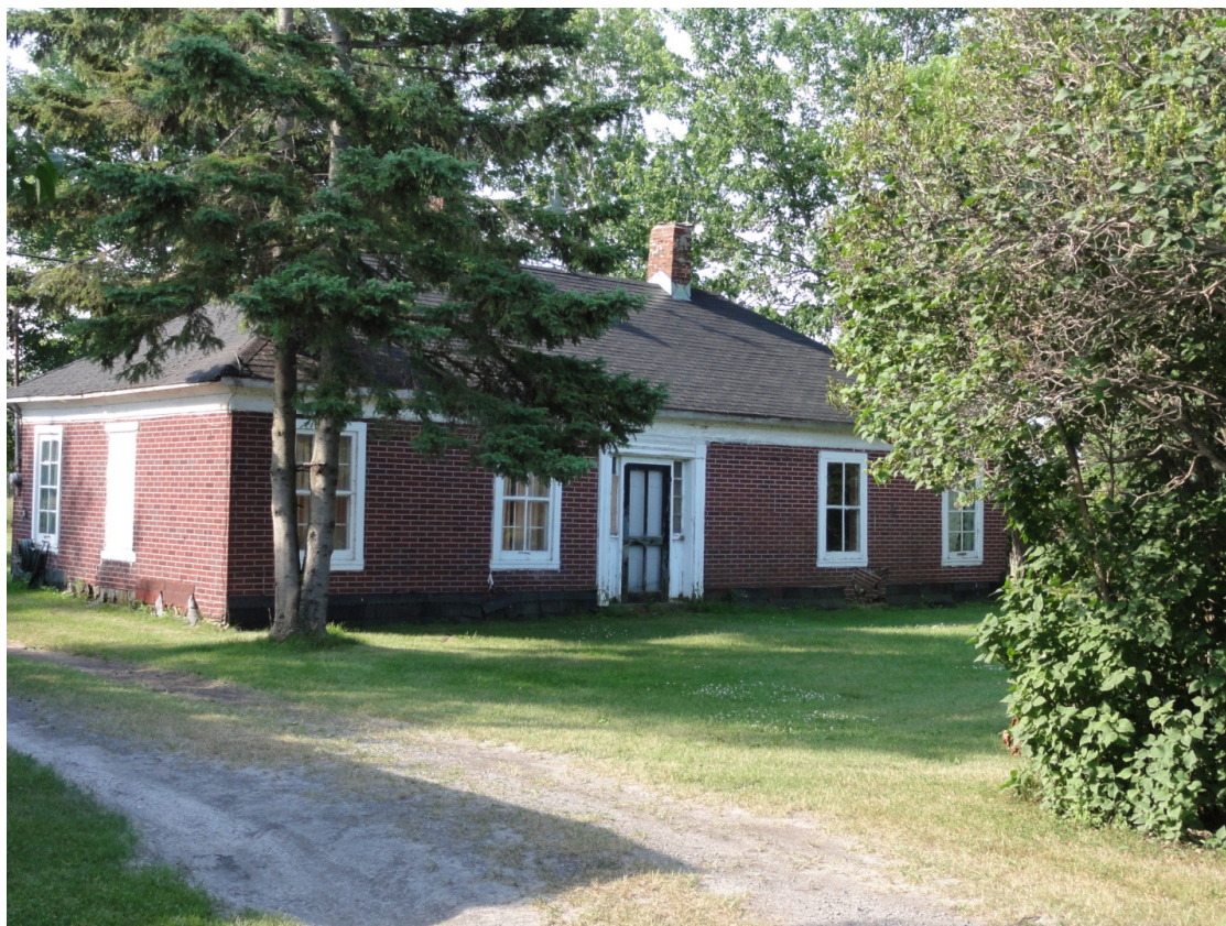
Plate 10: 12405 Front Road, BHR 8
