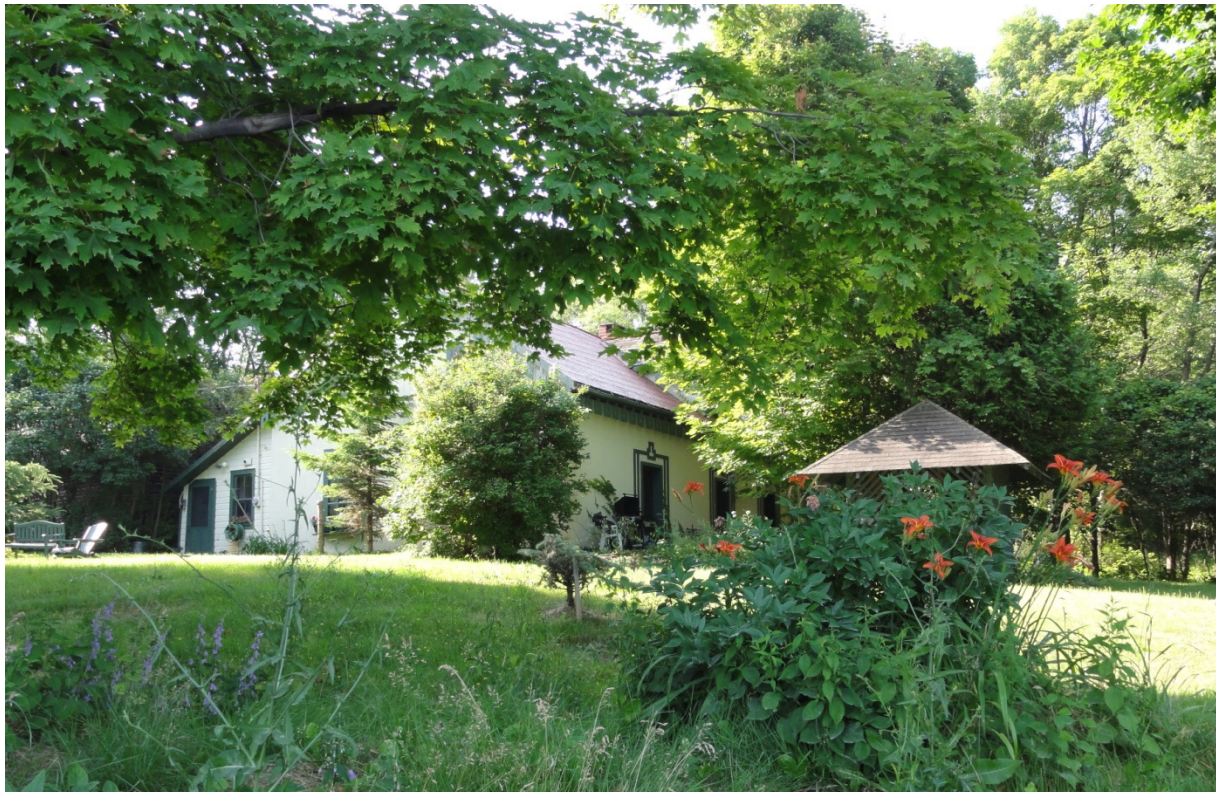
Plate 20: 14005 Front Road, BHR 15
