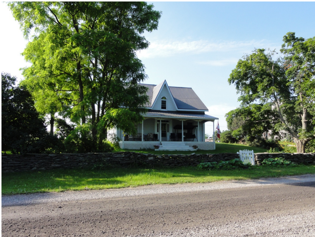
Plate 15: 12675 Front Road, BHR 11
