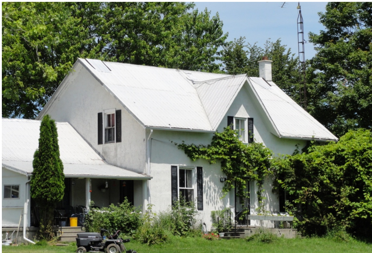
Plate 2: 2090 South Shore Road, BHR 2
