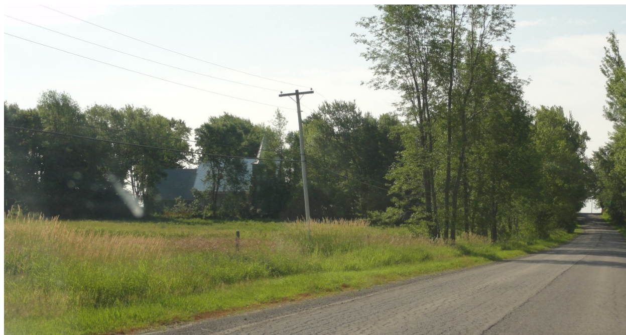
Plate 45: St. Paul’s Presbyterian Church, CHL 3, viewed from the north
