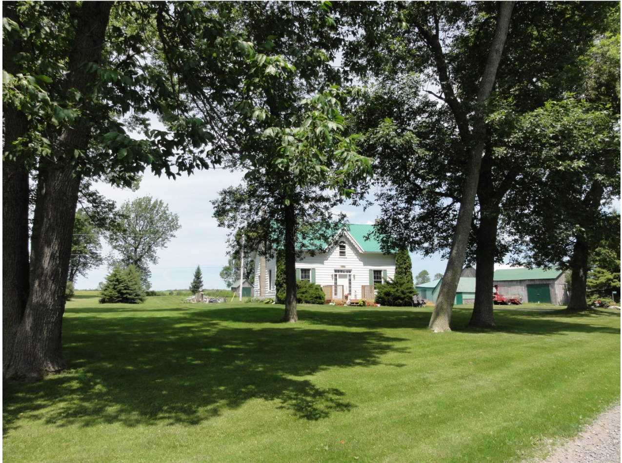
Plate 4: 3500 South Shore Road, BHR 4
