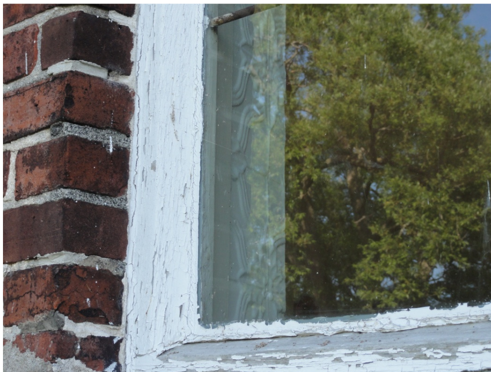
Plate 14: Detail of windows, St. Bartholomew's Catholic Church, BHR 10
