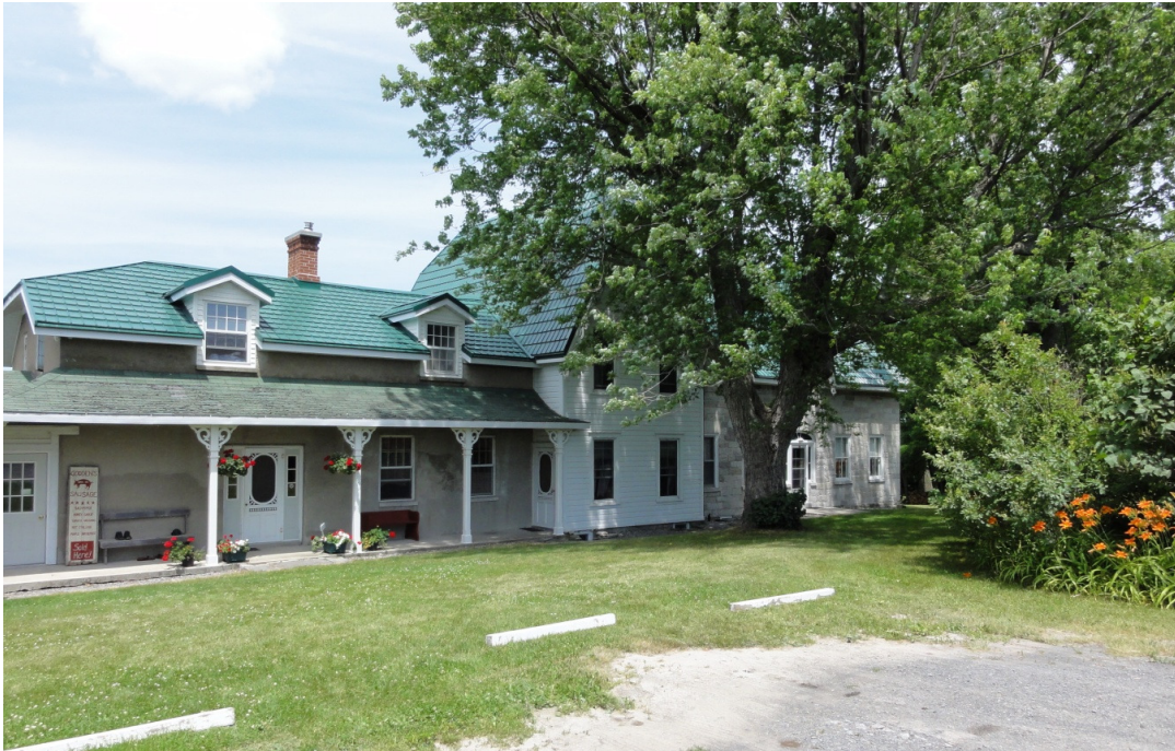
Plate 7: 3190 Front Road, BHR 7
