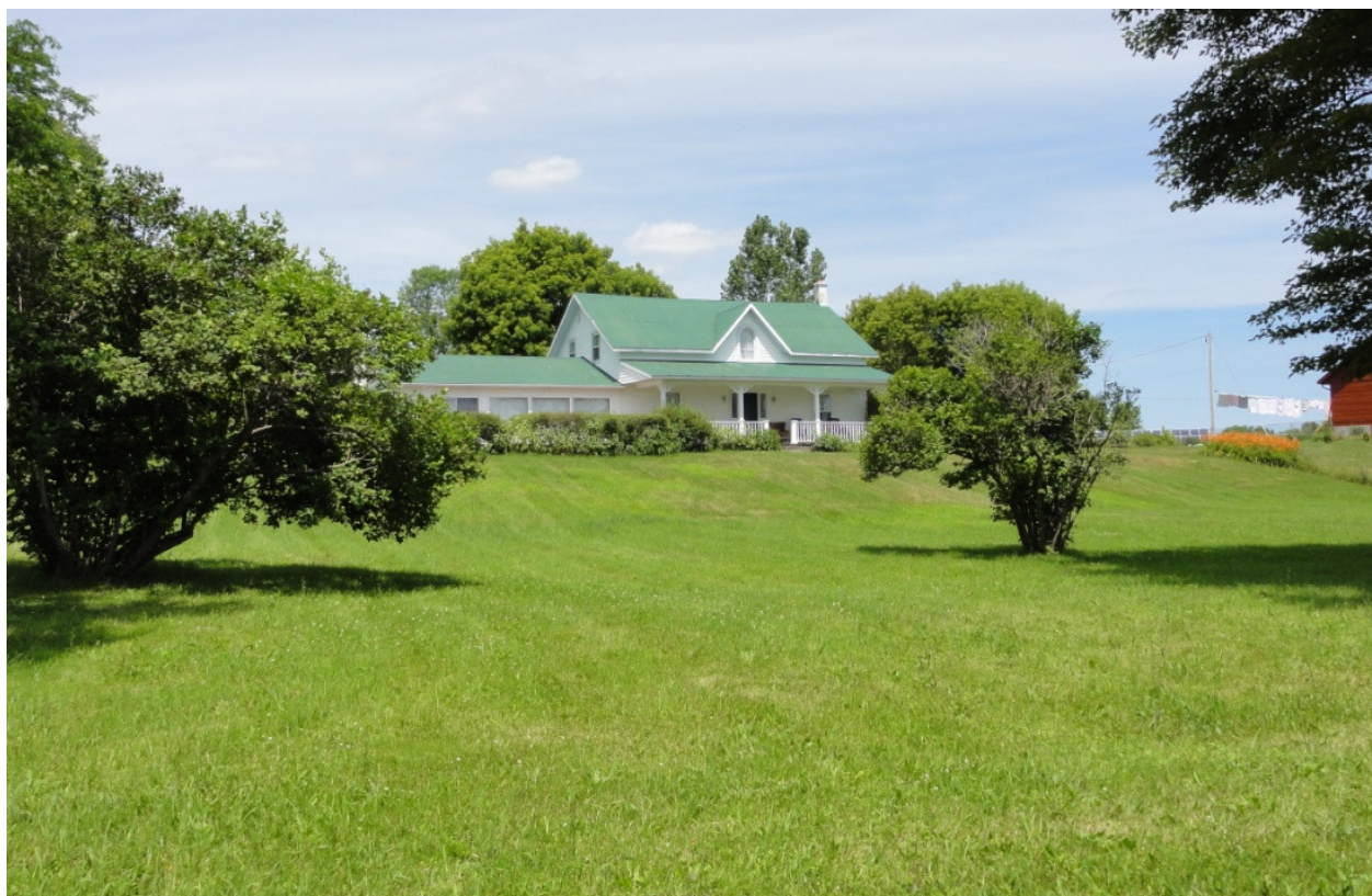
Plate 3: 2450 South Shore Road, BHR 3
