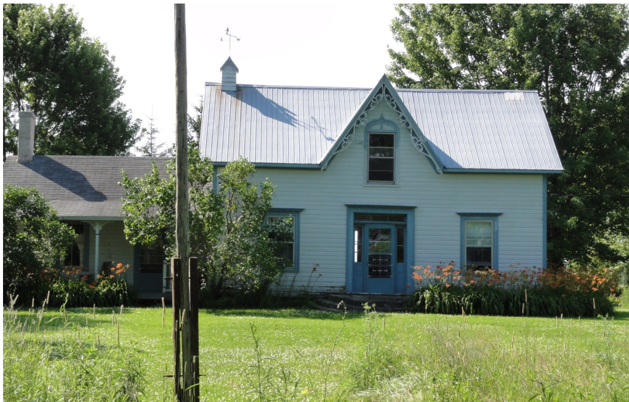
Plate 31: 4725 Second Concession Road, BHR 20
