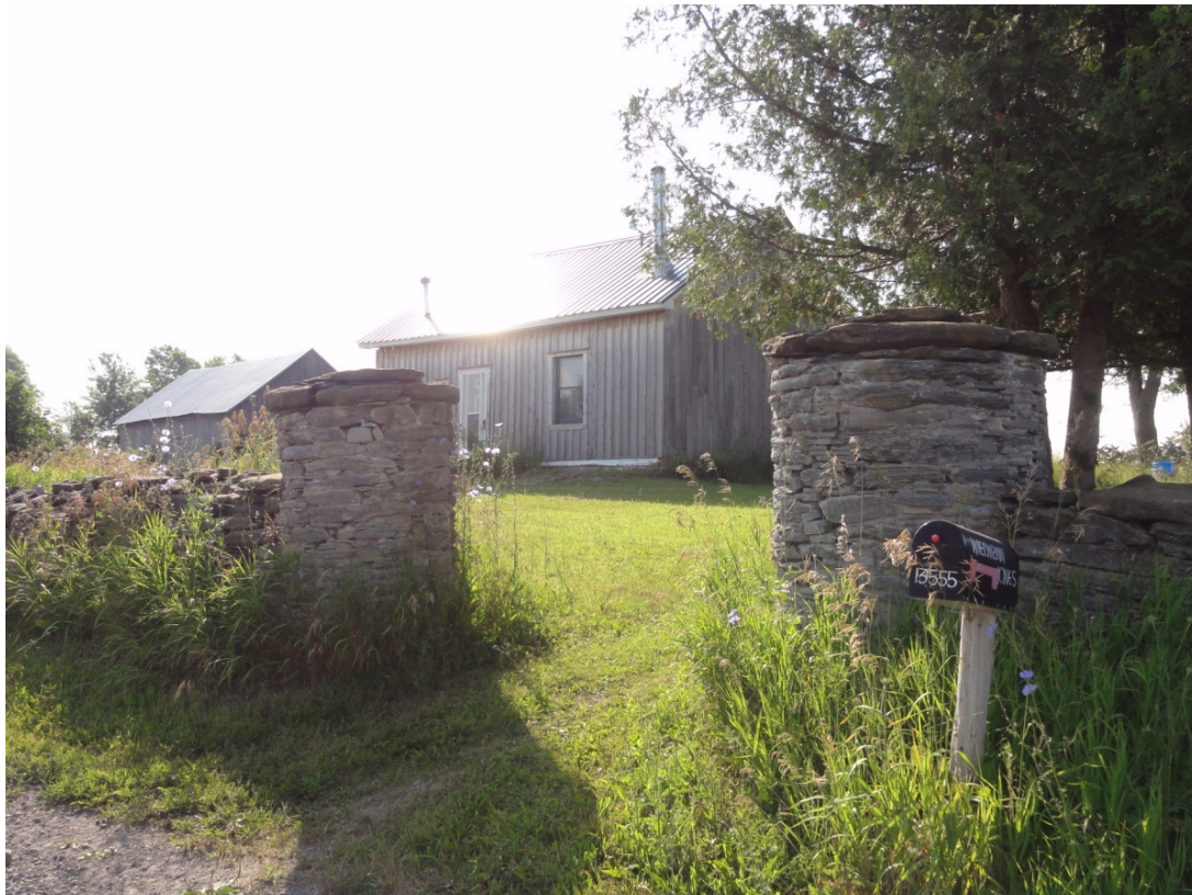
Plate 17: 13555 Front Road, BHR 13
