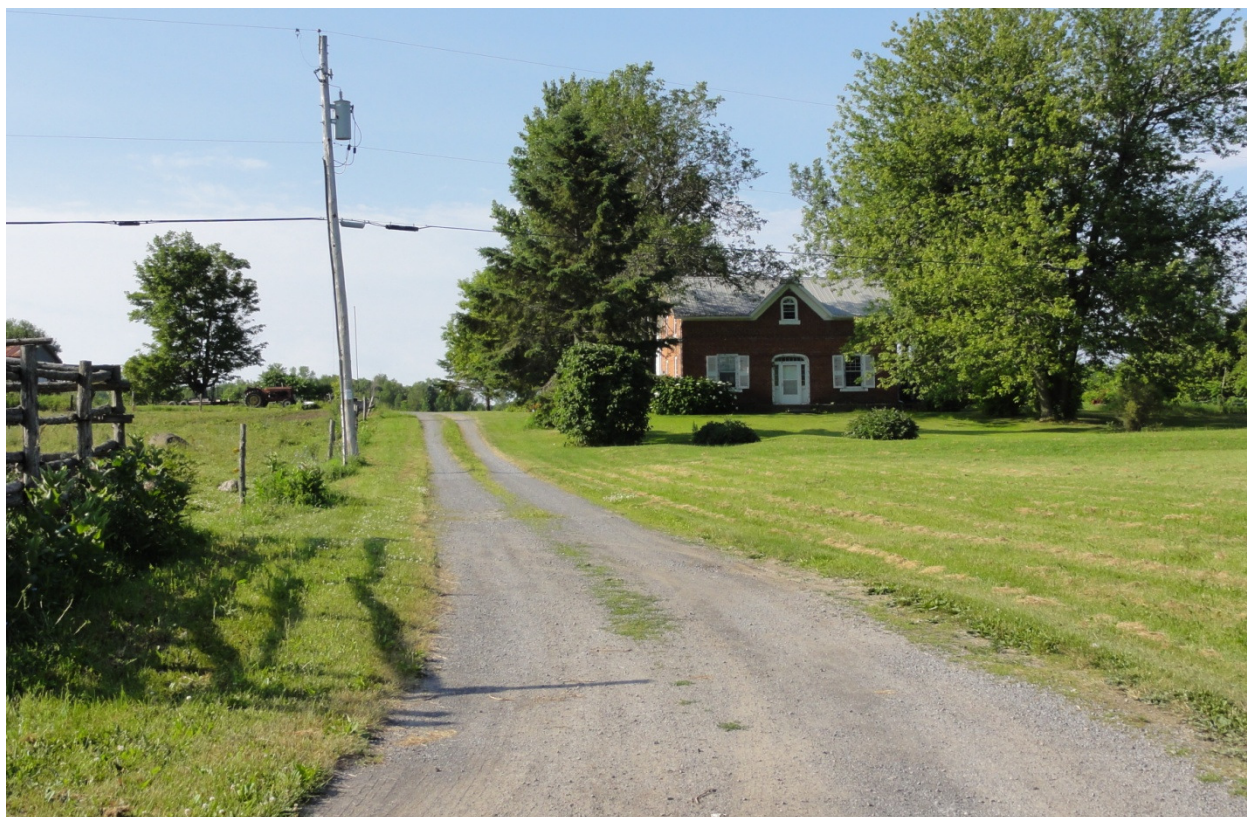
Plate 16: 12945 Front Road, BHR 12
