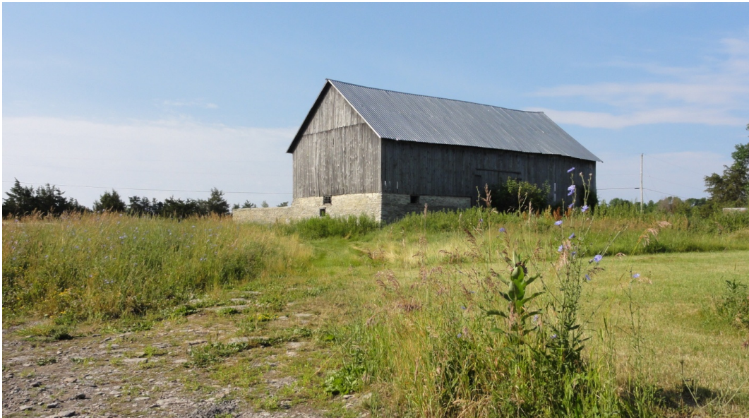
Plate 18: Barn at 13555 Front Road
