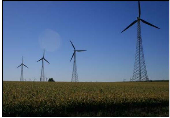
212 turbines visible from all orientations, nearest 0.4 miles (IABV)
