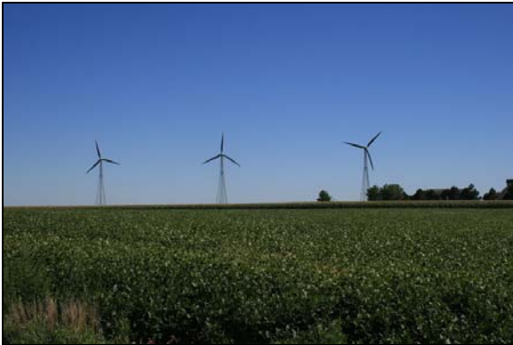
90 turbines visible from all orientations, nearest 0.6 miles (IABV)
