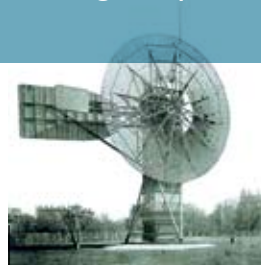
1888: Charles Brush develops first large wind generator producing 12 kW DC
