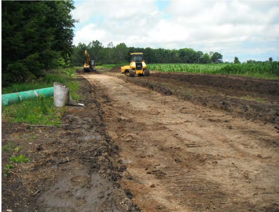
Photo 3 Typical access road construction at a wind project
