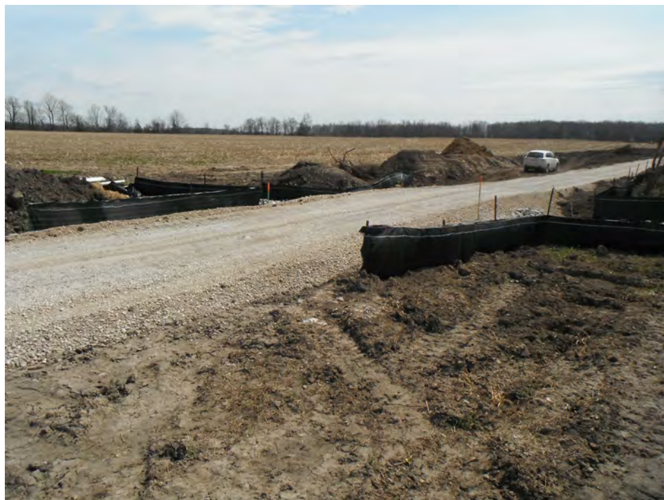
Photo 2 Typical access road construction at a wind project
